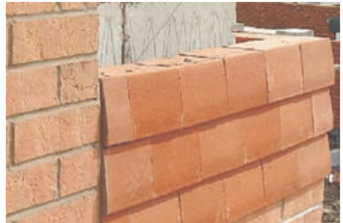
Protect brickwork from the elements
