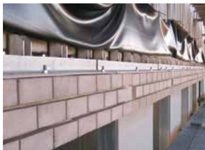
Fixing bracket details
