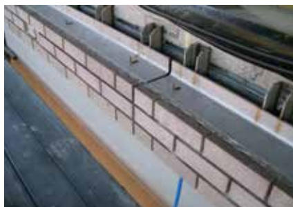
Fixing bracket details
