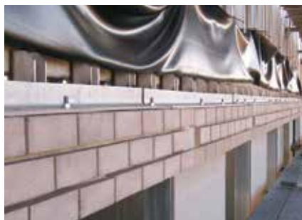
Fixing bracket details
